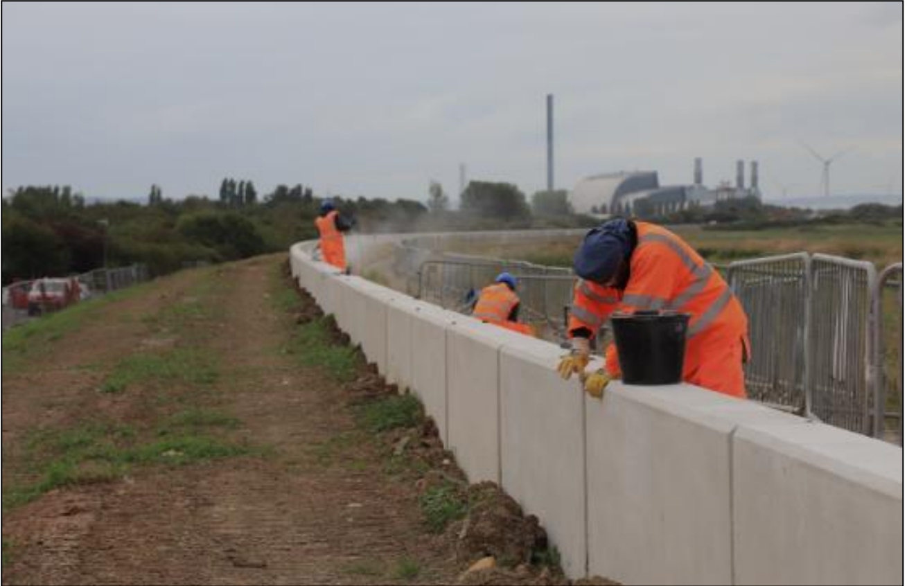
Plate A.2 Precast concrete flood wall 7
